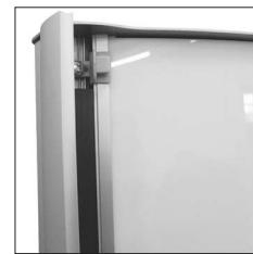
• Fix the other side of Opak Plexy by pushing it bottom-up. Be sure that opak plexi fits the channels well.
