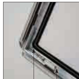
Sealing rubber Water drainage holes
